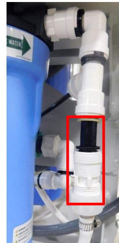
Figure 7. Part Number: ZI10124 AquaC Connection Kit - 3/4" GHT
